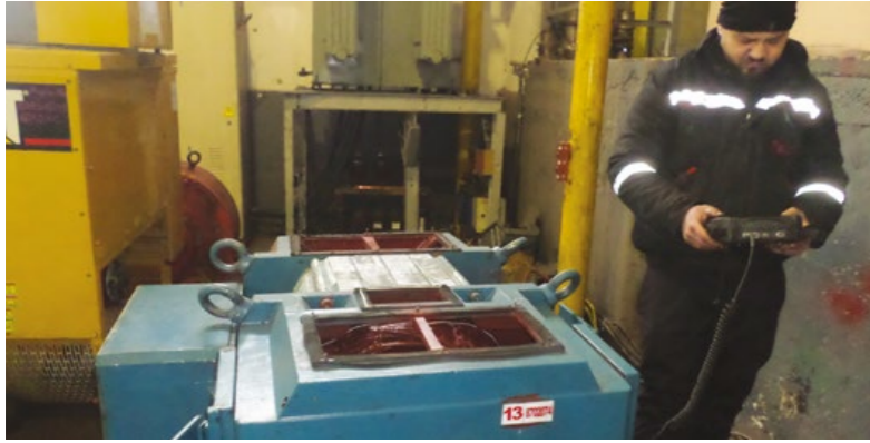
700 kW DC roller motor maintenance.
