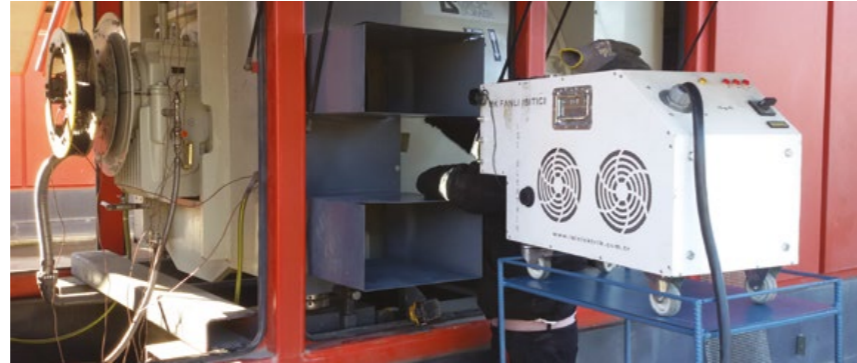
Tuzla purification 4360 kW Generator field maintenance.
