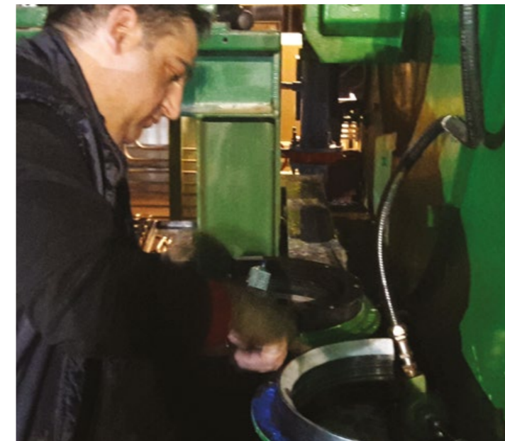
Our 15000 KVA generator field expertise operation.
