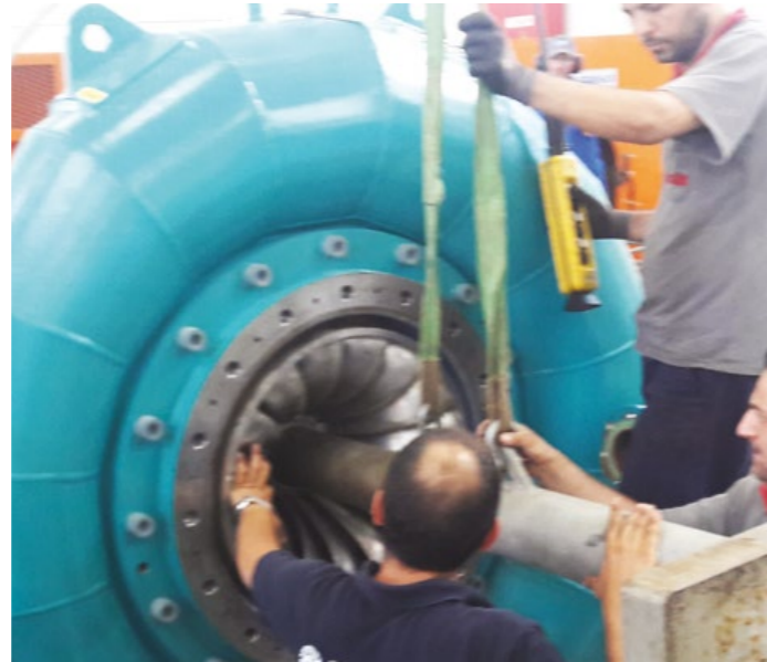
Our turnkey maintenance and repair work with 1400 KW Hydrogen generator Workshop and field service.
